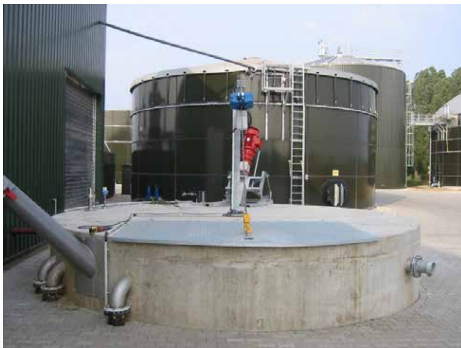
Figure 6.2: Storage for liquid feedstock (Fachverband Biogas e.V.)
